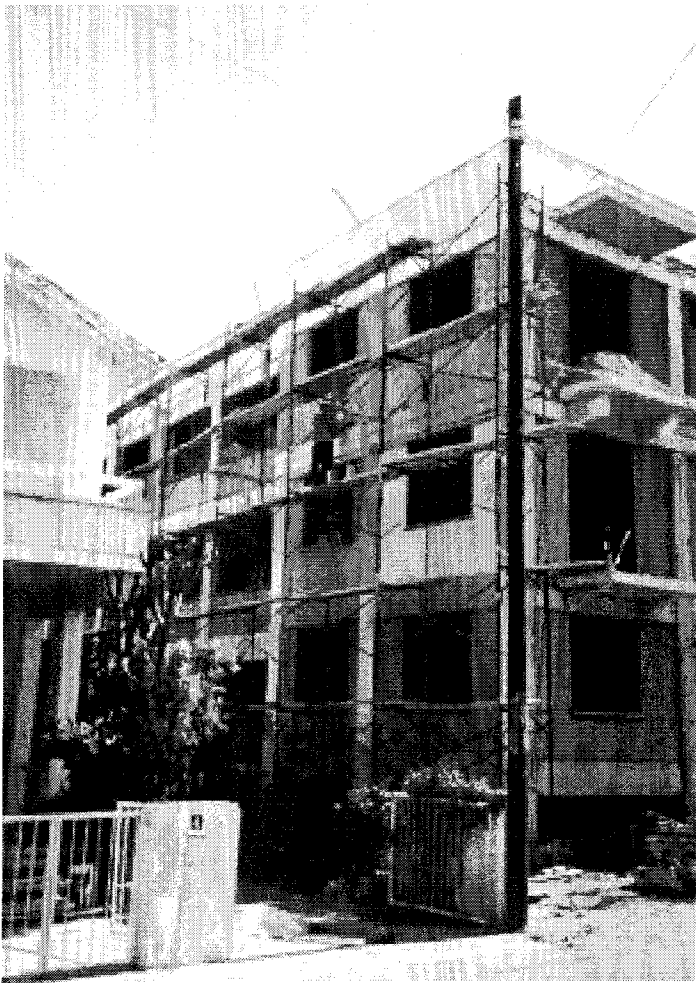
Fig. 9. Color testing on the east side of the building.
